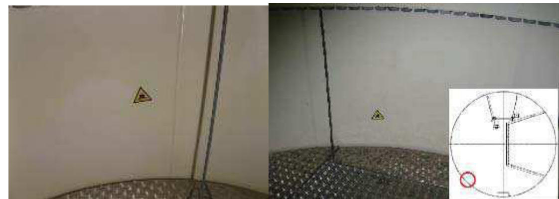
Figure 2.2.2: “Max Load on Platform 1t” (item 208014) Place the signs approximately 30 cm above the platform, opposite the ladder/lif as shown in the inserted drawing
