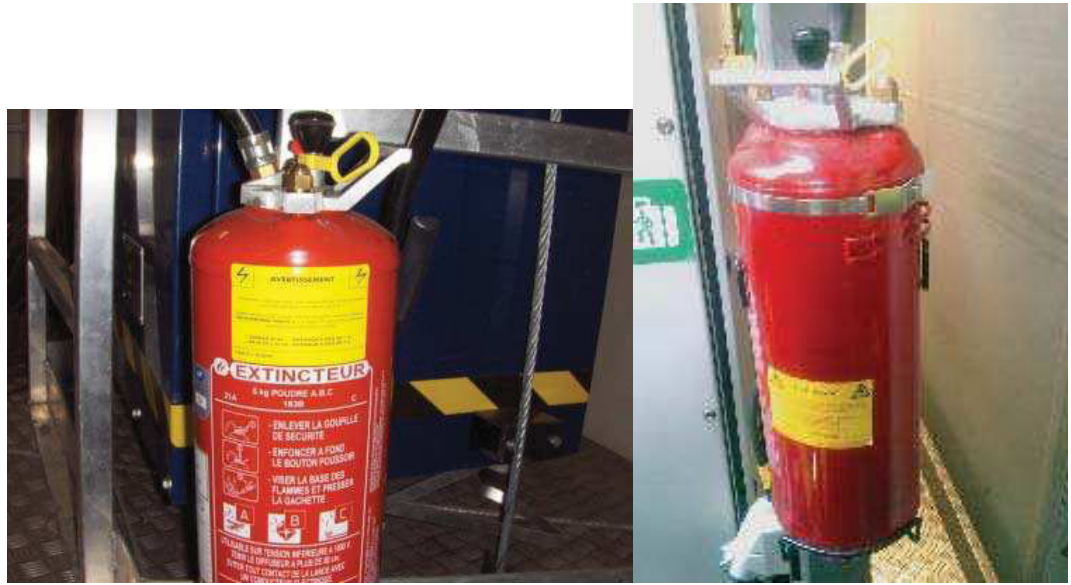
Figure 4.1: “Electrical Risk” Place the signs on the two extinguishers (bottom and nacelle)
