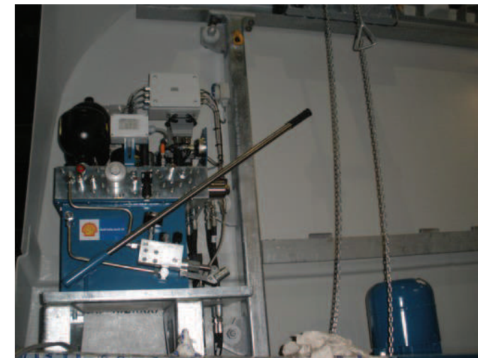
Fig. 83 Hydraulic unit for rotor brake and yaw brakes
