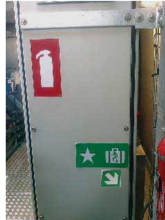
Figure 3.2.6: “Rescue Equipment / Arrow” (item 208020/208021) and “Fire Extinguisher” (item 208007) Place the signs on the end cover of the nacelle controller
