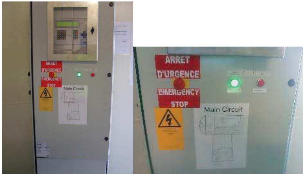
Figure 2.1.3: “Emergency stop / Arrêt d’urgence”, “Caution ! Battery voltage remains on after deenergizing” (item 119077) and his translation, “Main circuit” (item 119081), Place the signs on the ground controller
