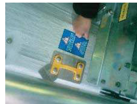
Figure 3.3: “Don’t use anchorage point for the emergency evacuation system” Place the sign near the anchorage point at the rear of the internal crane.
