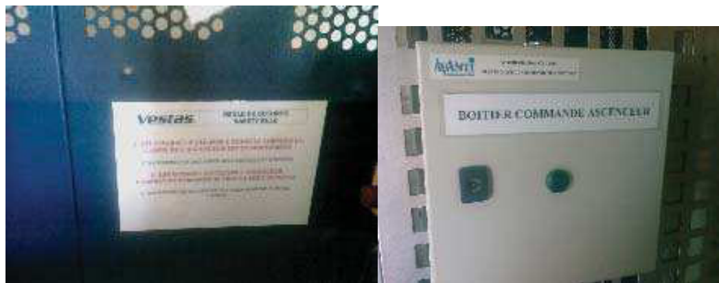
Figure 2.1.8: “Safety rule Ladder/Service lift” Place the sign inside the service lift “Boitier de commande ascenseur” Plan the sign outside the service lift
