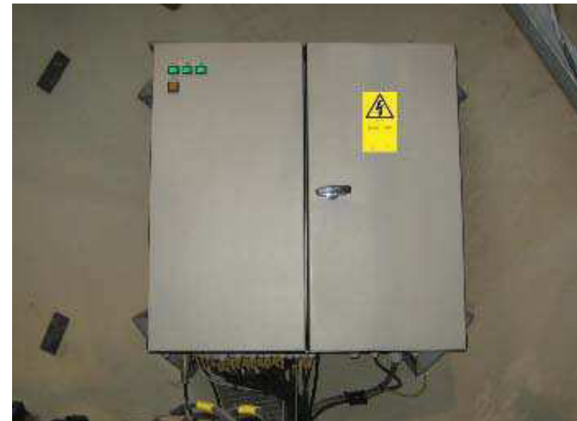
Figure 3.4.5: “Hub controller” (item 119075) Place the sign in the center of the upper part on the right cabinet door on the hub controller
