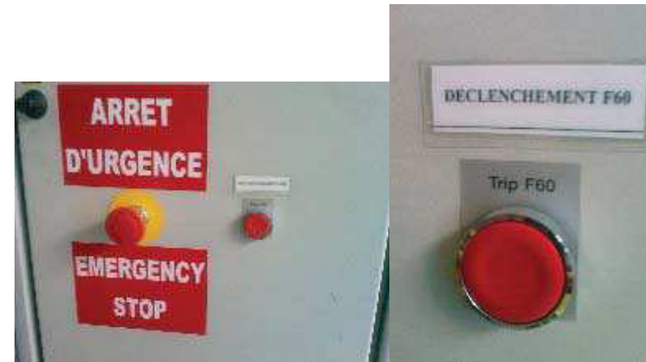
Figure 3.2.2 “Emergency stop / Arrêt d’urgence”, “Declenchement F60” Place the signs around the button on the controller
