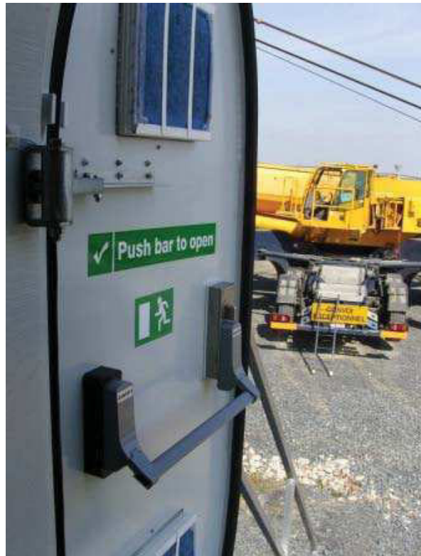
Figure 2.1.2: “Emergency Exit” (item 208011), “Push bar to open” and his translation Place the signs on the upper part of the tower door
