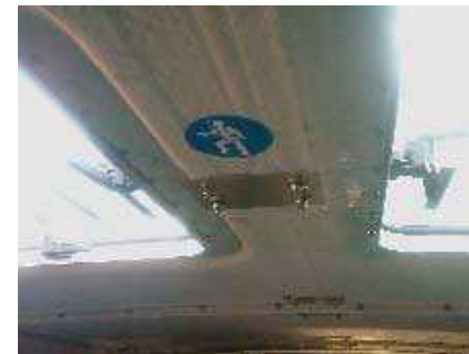
Figure 3.2: “Safety Harness Required” (Item 208006) Place the sign next to each skylight on the inside of the roof.
