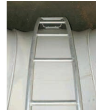
Fig. 74 Hub ladder in position
